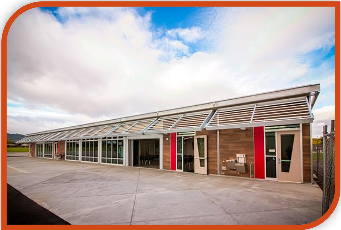
Gen7 STEAM Modular Classrooms—open to the outside
