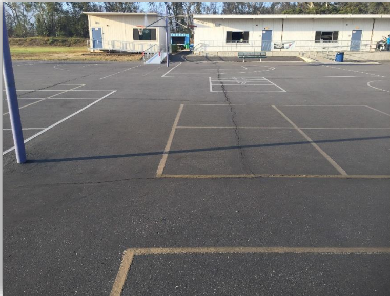
ELLWOOD ELEMENTARY AREA B - PHOTO 11
