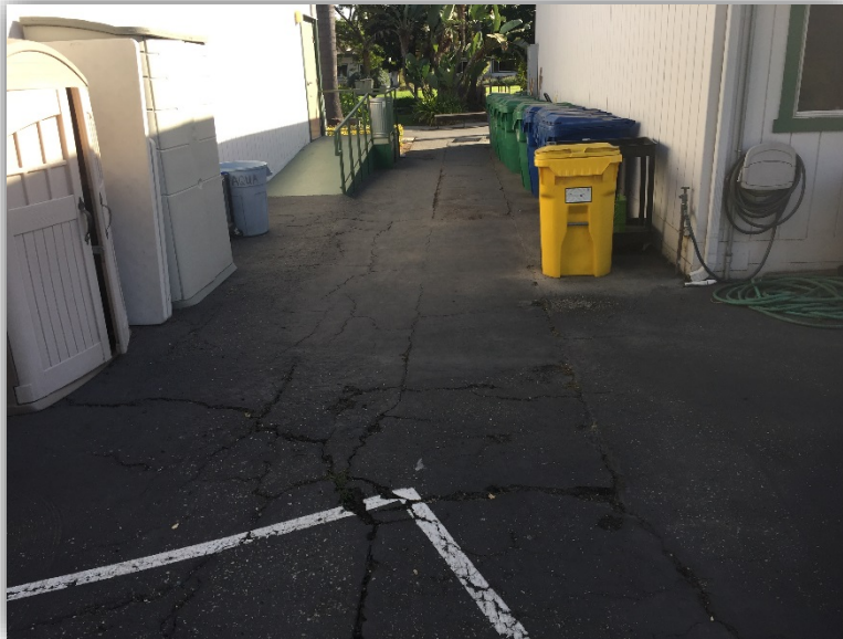
DISTRICT OFFICE AREA F - PHOTO 9
