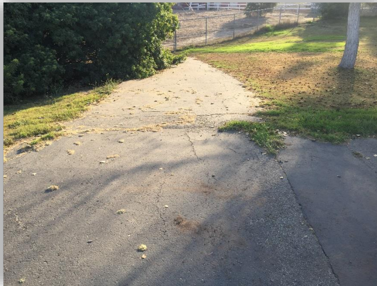
ISLA VISTA ELEMENTARY AREA C - PHOTO 12
