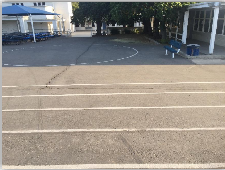
ELLWOOD ELEMENTARY AREA B - PHOTO 7
