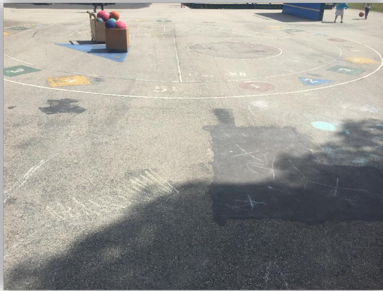
MOUNTAIN VIEW ELEMENTARY AREA C - PHOTO 1
