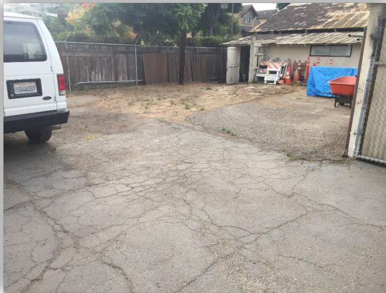
MAINTENANCE & TRANSPORTATION AREA B - PHOTO 3
