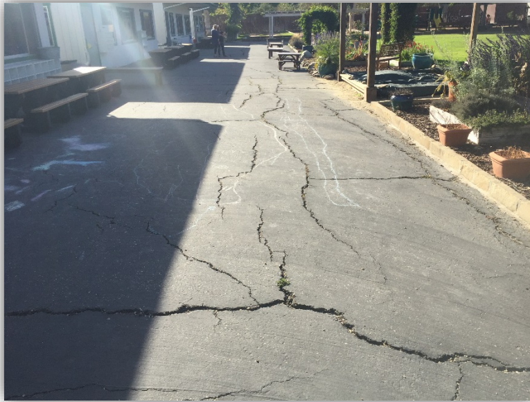
DISTRICT OFFICE AREA F - PHOTO 3
