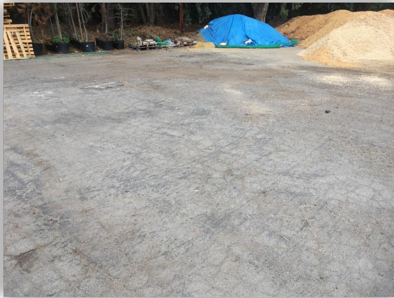
MAINTENANCE & TRANSPORTATION AREA B - PHOTO 8
