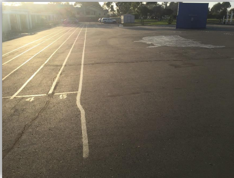
ELLWOOD ELEMENTARY AREA B - PHOTO 9
