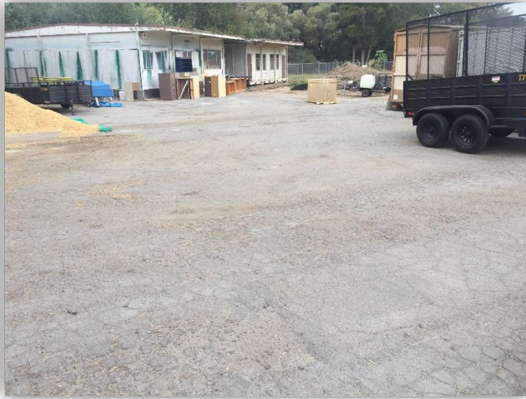
MAINTENANCE & TRANSPORTATION AREA B - PHOTO 9
