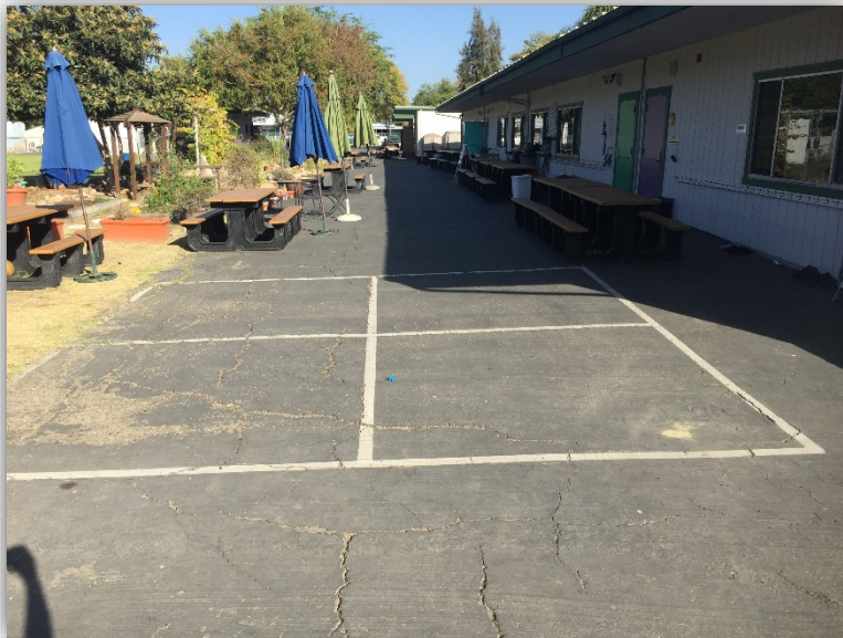
DISTRICT OFFICE AREA F - PHOTO 8
