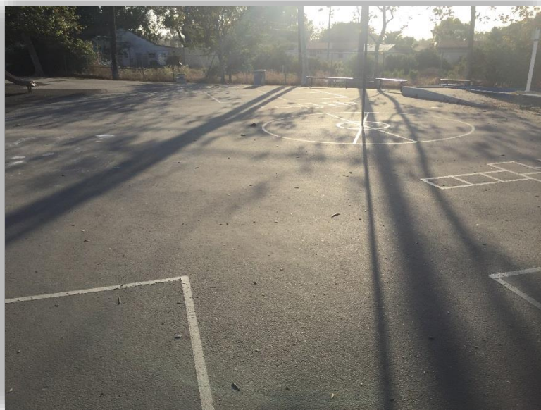
ISLA VISTA ELEMENTARY AREA C - PHOTO 4
