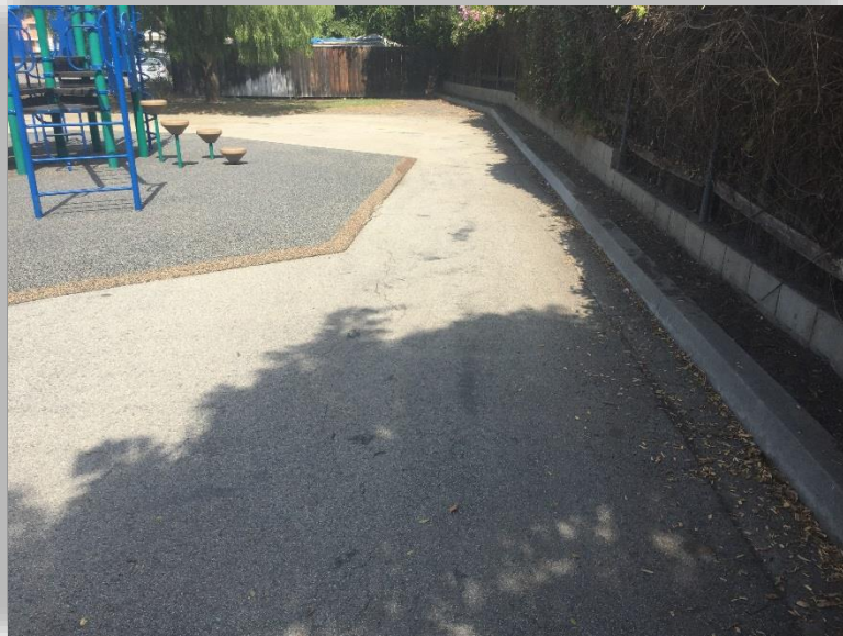
MOUNTAIN VIEW ELEMENTARY AREA C - PHOTO 4
