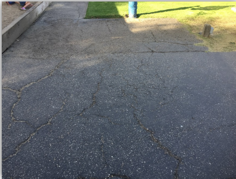
DISTRICT OFFICE AREA F - PHOTO 4
