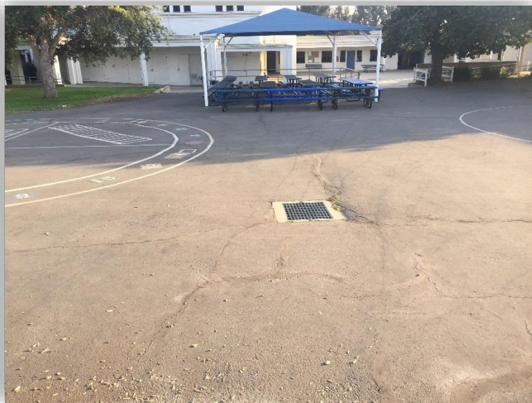
ELLWOOD ELEMENTARY AREA B - PHOTO 8
