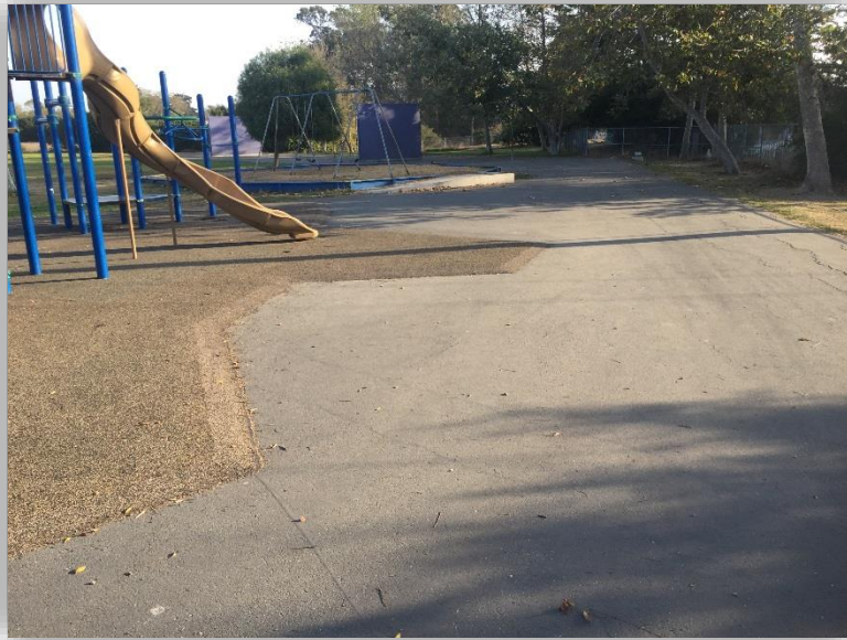
ISLA VISTA ELEMENTARY AREA C - PHOTO 7
