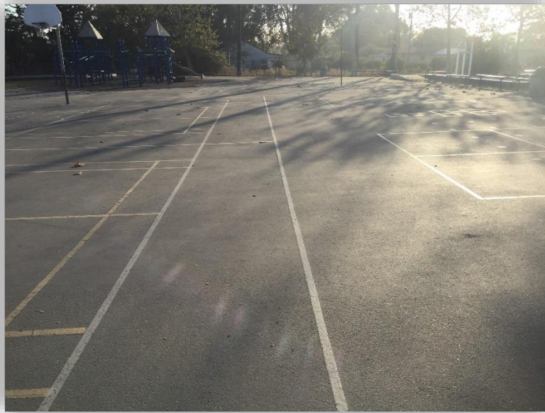
ISLA VISTA ELEMENTARY AREA C - PHOTO 3
