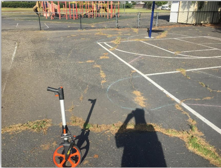
BRANDON ELEMENTARY AREA C - PHOTO 2
