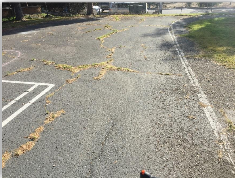
BRANDON ELEMENTARY AREA C - PHOTO 1
