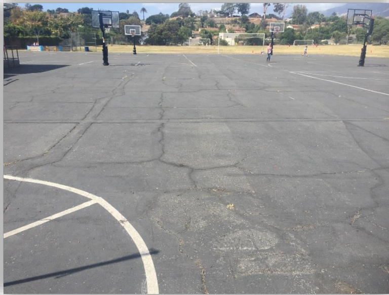
MOUNTAIN VIEW ELEMENTARY AREA B - PHOTO 2
