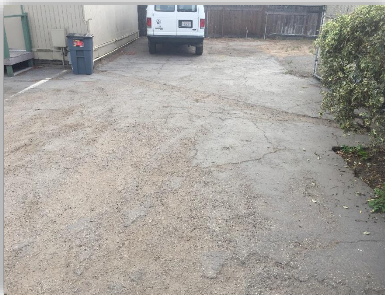
MAINTENANCE & TRANSPORTATION AREA B - PHOTO 2
