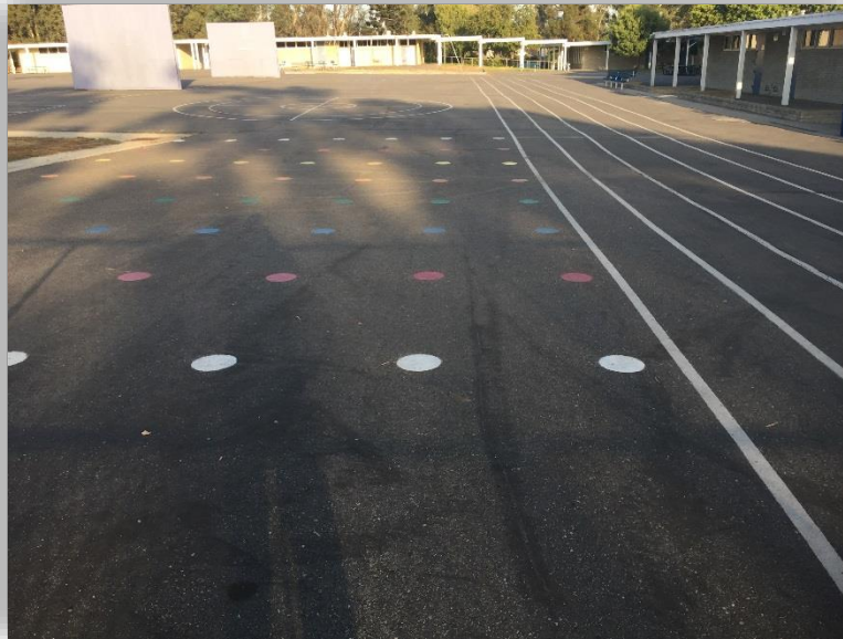
ELLWOOD ELEMENTARY AREA B - PHOTO 1
