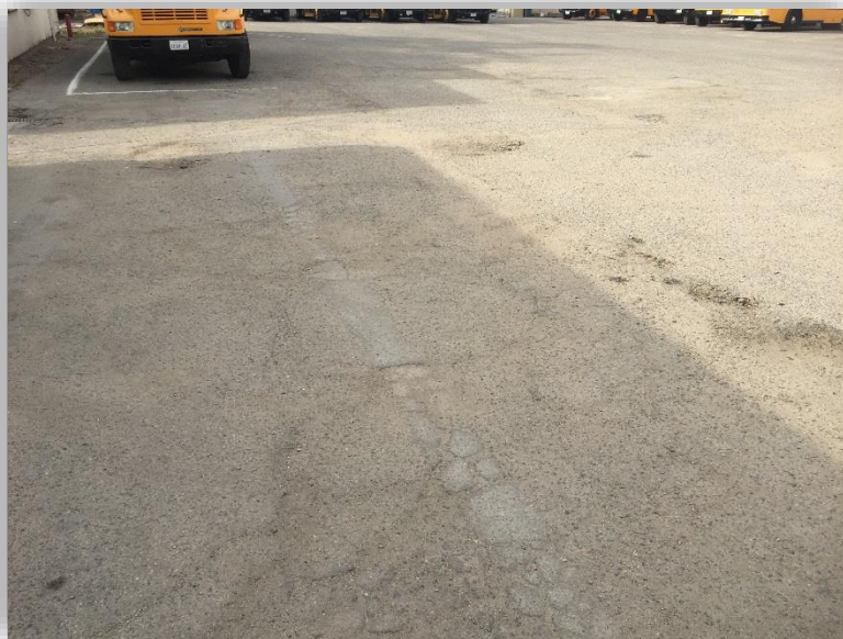
MAINTENANCE & TRANSPORTATION AREA B - PHOTO 10
