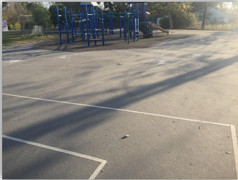
ISLA VISTA ELEMENTARY AREA C - PHOTO 5
