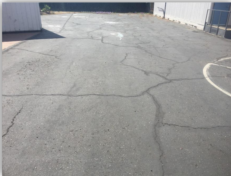
MOUNTAIN VIEW ELEMENTARY AREA B - PHOTO 1
