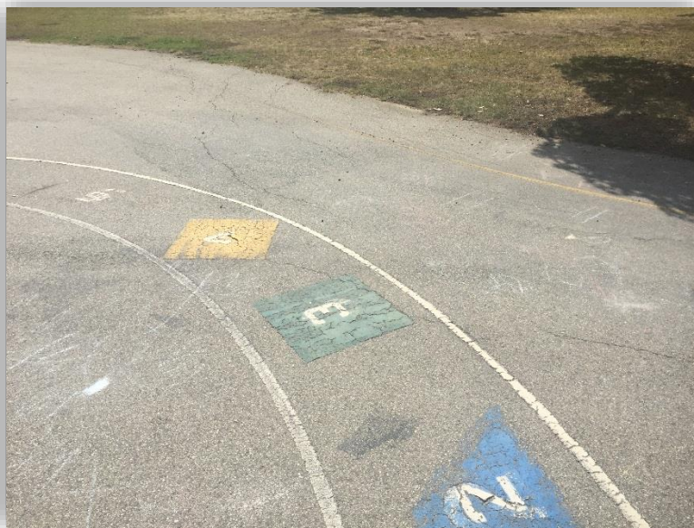
MOUNTAIN VIEW ELEMENTARY AREA C - PHOTO 2
