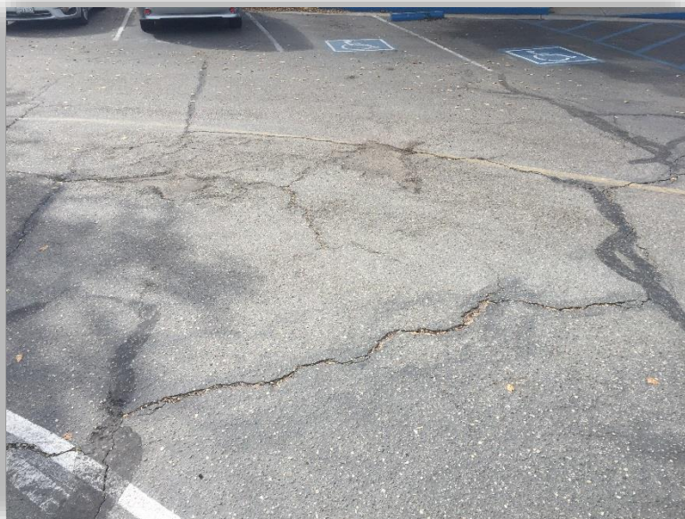
MOUNTAIN VIEW ELEMENTARY AREA A - PHOTO 4
