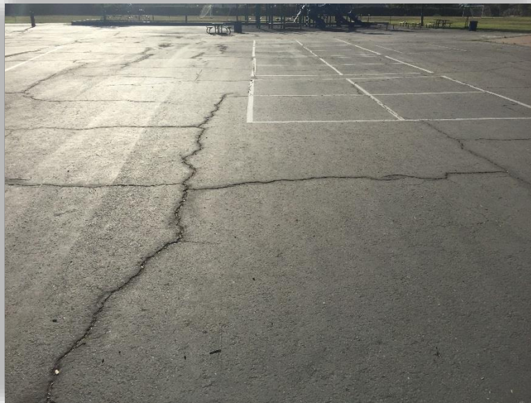
BRANDON ELEMENTARY AREA C - PHOTO 3
