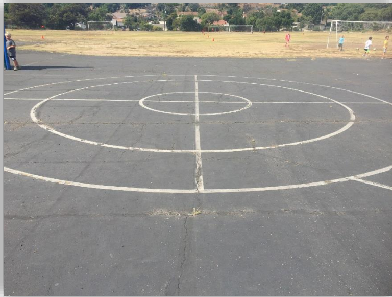
MOUNTAIN VIEW ELEMENTARY AREA B - PHOTO 5
