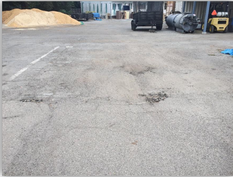
MAINTENANCE & TRANSPORTATION AREA B - PHOTO 7
