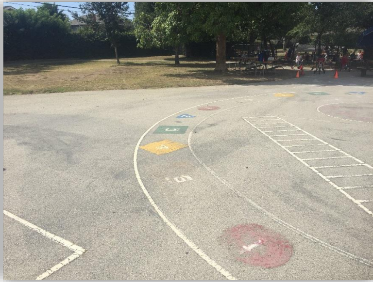
MOUNTAIN VIEW ELEMENTARY AREA C - PHOTO 3
