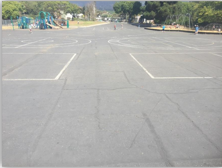
MOUNTAIN VIEW ELEMENTARY AREA B - PHOTO 4
