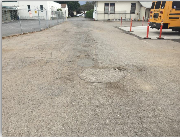
MAINTENANCE & TRANSPORTATION AREA B - PHOTO 5
