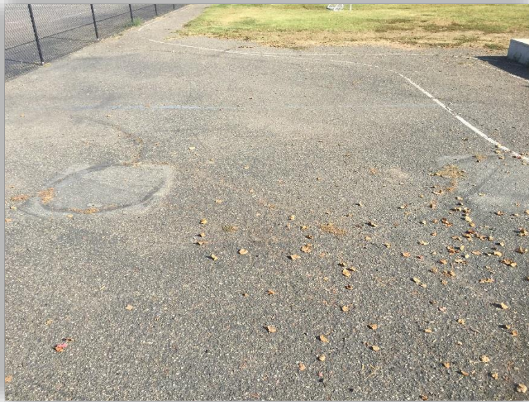
BRANDON ELEMENTARY AREA C - PHOTO 4
