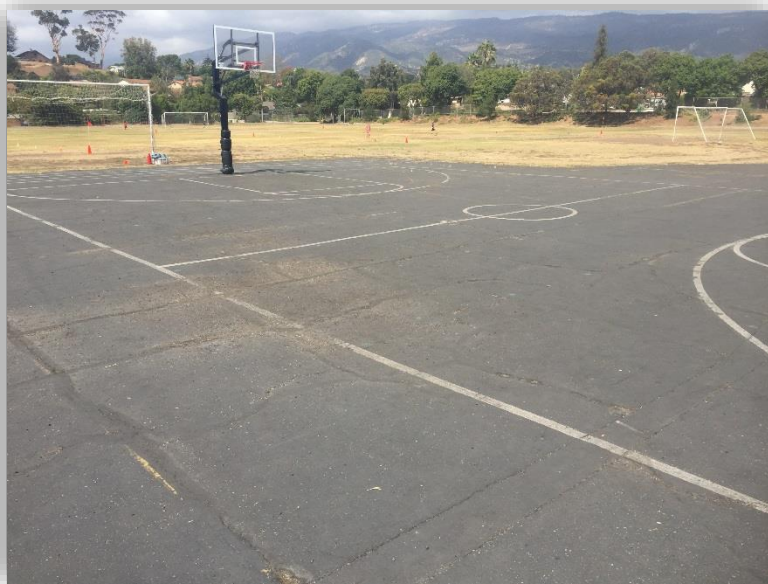
MOUNTAIN VIEW ELEMENTARY AREA B - PHOTO 3
