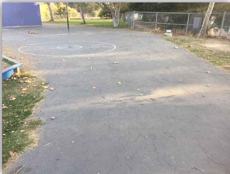
ISLA VISTA ELEMENTARY AREA C - PHOTO 8
