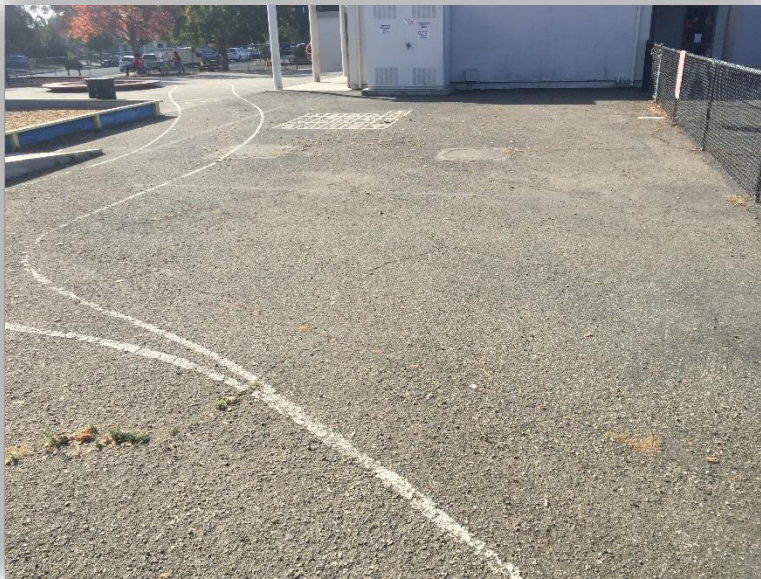
BRANDON ELEMENTARY AREA C - PHOTO 3
