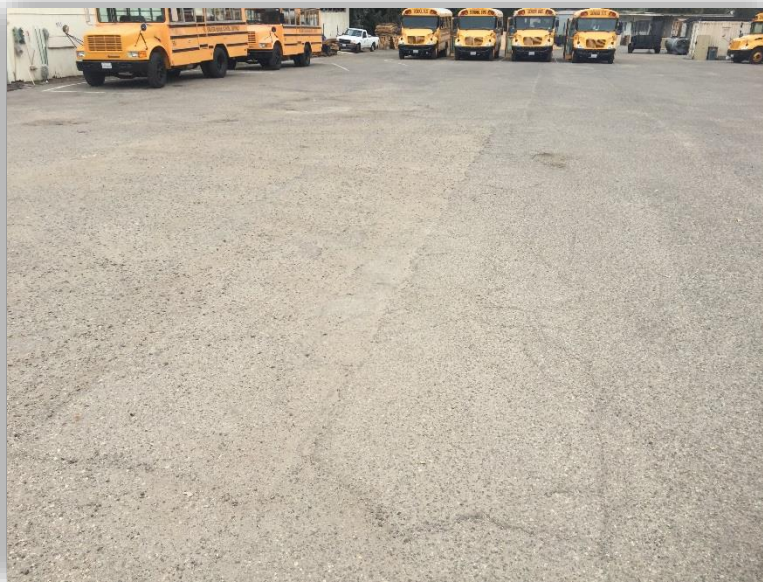
MAINTENANCE & TRANSPORTATION AREA B - PHOTO 6
