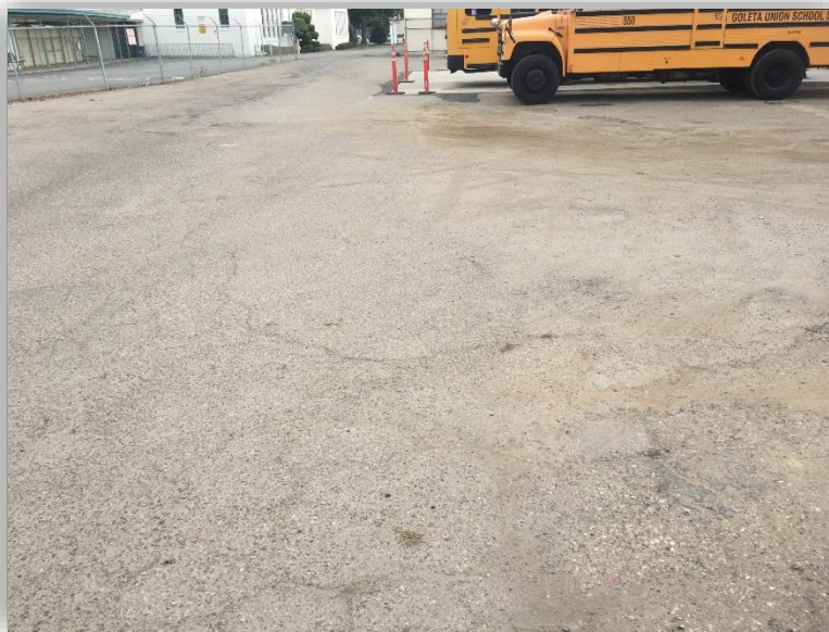
MAINTENANCE & TRANSPORTATION AREA B - PHOTO 4
