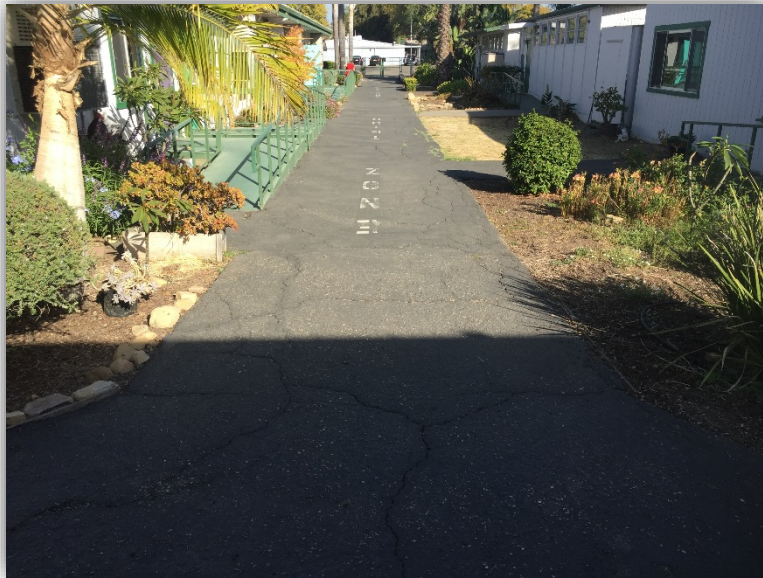
DISTRICT OFFICE AREA F - PHOTO 7
