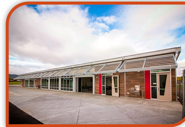
Gen7 STEAM Modular Classrooms—open to the outside
